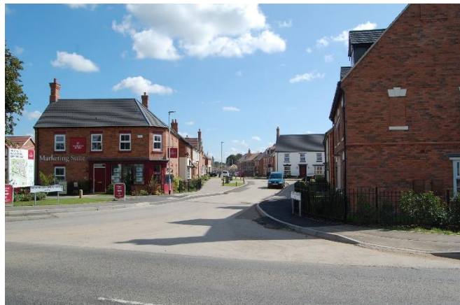
FIGURE 15: BARLEY FIELDS UNDER-CONSTRUCTION
