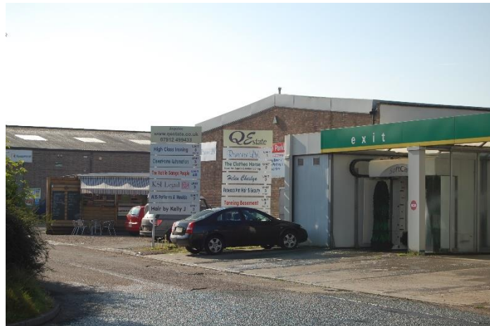
FIGURE 20: QUENIBOROUGH INDUSTRIAL ESTATE
