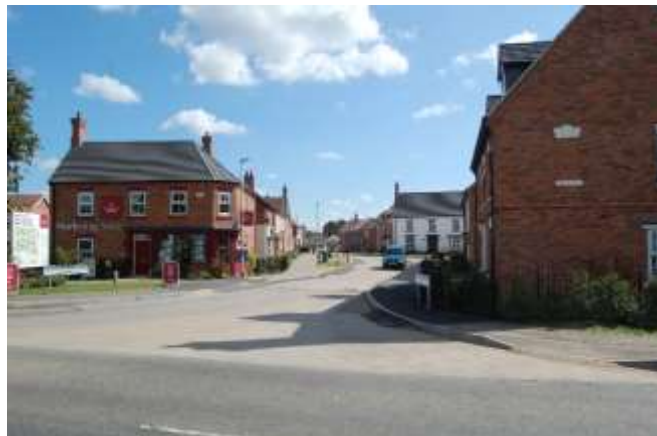
FIGURE 15: BARLEY FIELDS UNDER-CONSTRUCTION
