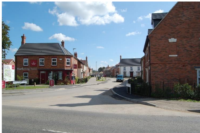
FIGURE 16: BARLEY FIELDS UNDER-CONSTRUCTION
